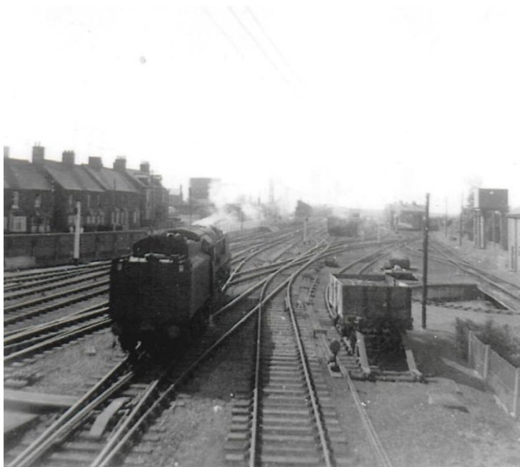
“Hotspur” photographed from the footbridge showing the massive tender and much of the railway infrastructure at Hunstanton. On the right is the turntable, water tower and engine shed. In the distance are the sidings where excursion trains were held until the return journey in the evening.
